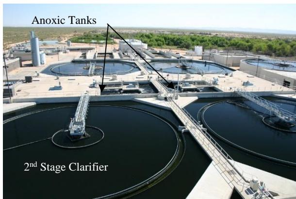
Figure 5 – 2<sup>nd</sup> Stage Anoxic Tanks & Clarifiers
